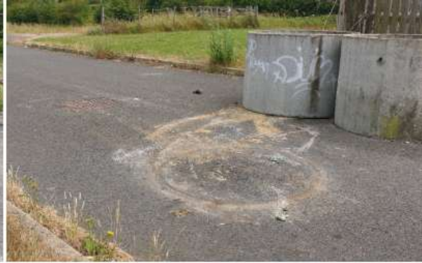
Rutledge Ave end of Southern Link Road
